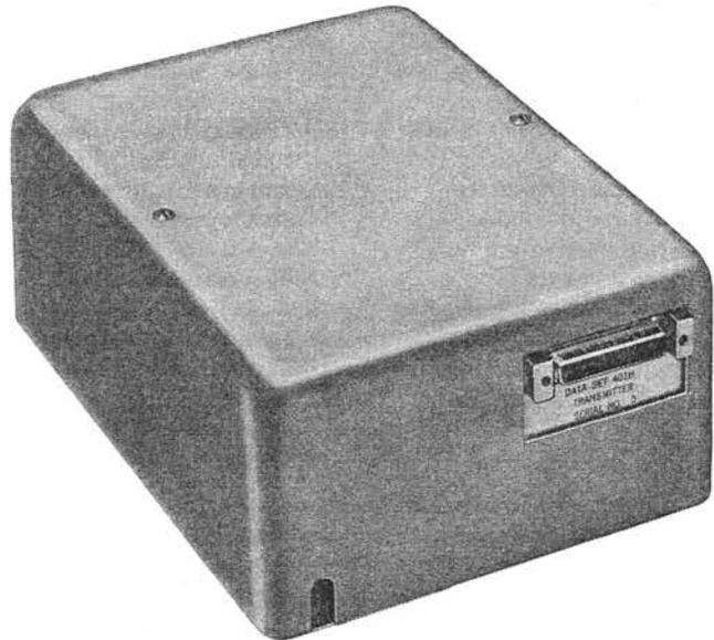
Each is an integrated set which combines a data transmitter, audible answer-back circuits, remote test circuits, and a telephone set in one housing. It is a low speed parallel transmitter in one direction delivering 3 to 14 frequency tones having a possibility of 99 different alphanumeric characters at a rate of 20 characters per second. Synchronization of timing is not required.
